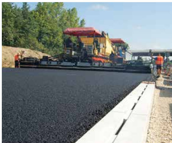
Figure 8: Paving SMA binder course
