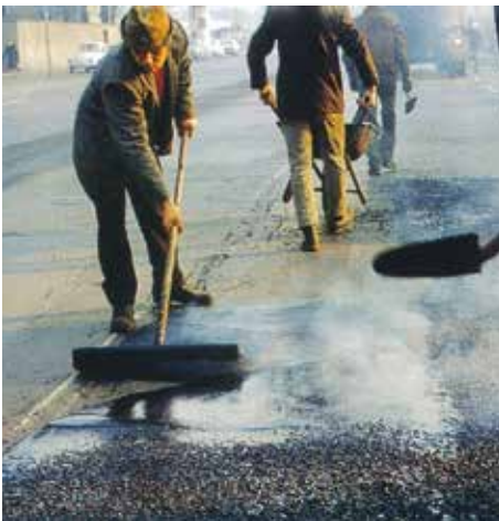
Figure 1: Paving an „asphalt mastic with a gritting“
